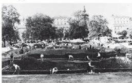
Digging air raid defences in London, September 1938.
