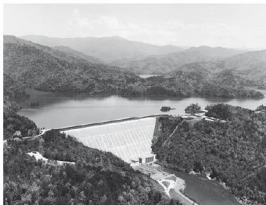
The Fontana Dam, one of the TVA's later projects. Dams such as these revitalised farmland, provided jobs and brought electric power to the area.
